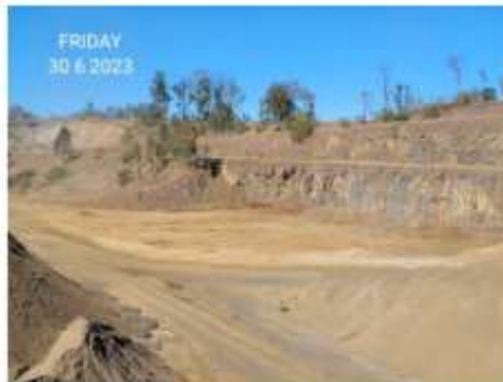
June 2023 – West Pit fill complete (looking east)
