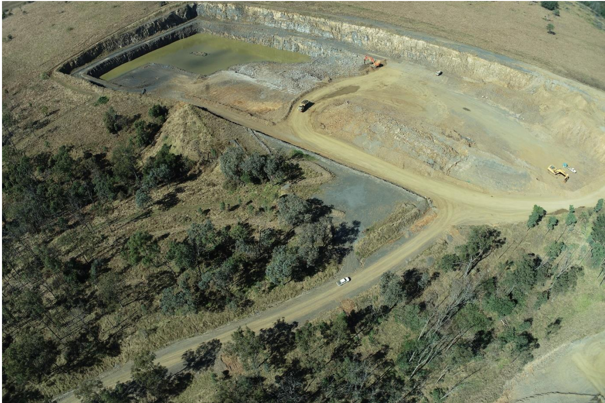
Figure 5 – Looking south-east across current east pit (Aerial July 2022)
